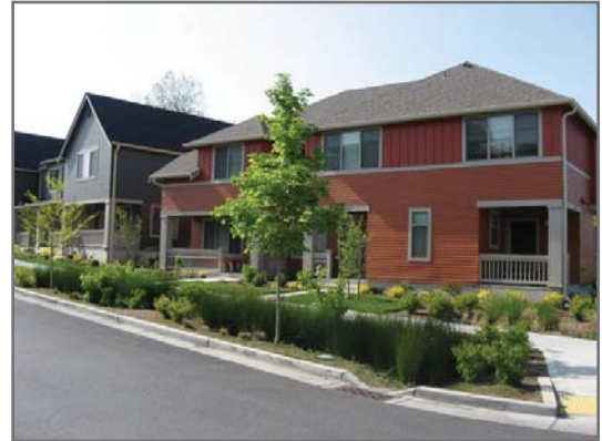
Swale Along Street with Curb Cut
