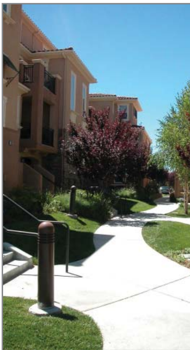
Bollard Lighting along Walkways
