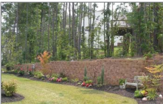
Landscaped Residential Retaining Wall
