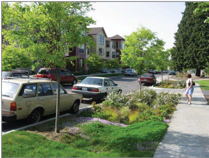
Sidewalk with Permeable Pavement and Adjacent to Bioswale
