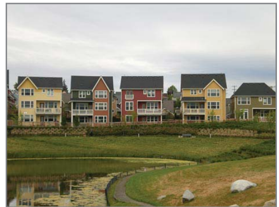
Neighborhood Bioretention Pond
