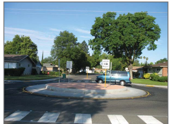
Mini Roundabout with Mountable Center Island
