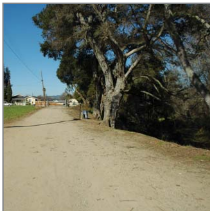
Corralitos Creek Embankment
