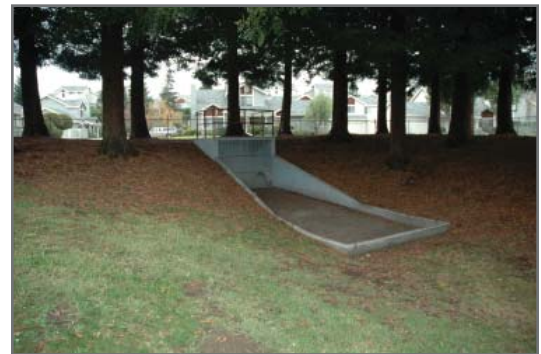
Existing Crestview Park Detention Basin
