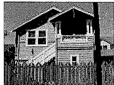
ABOVE: Desirable This is an alley view of a new accessory building that includes a secondary unit above a garage.
